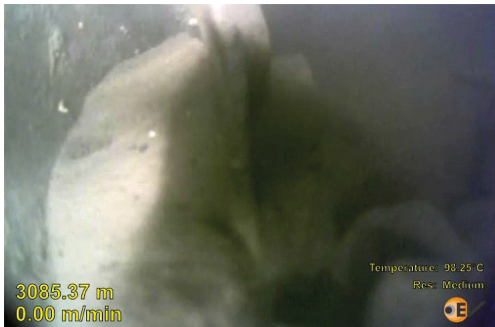
Figure 3: Downview image of obstruction believed to be collapsed liner
